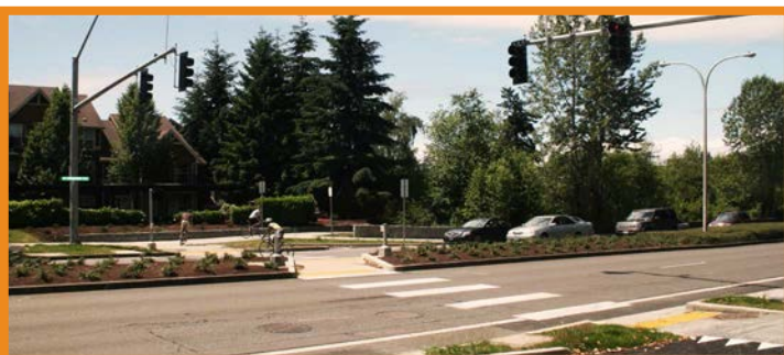
Photo: Evergreen Road Crossing, Washington County
