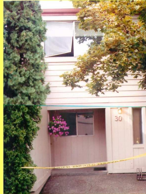
Window safety is not just an urban, high rise concern.
